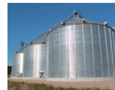
钢板仓 Steel Silo
